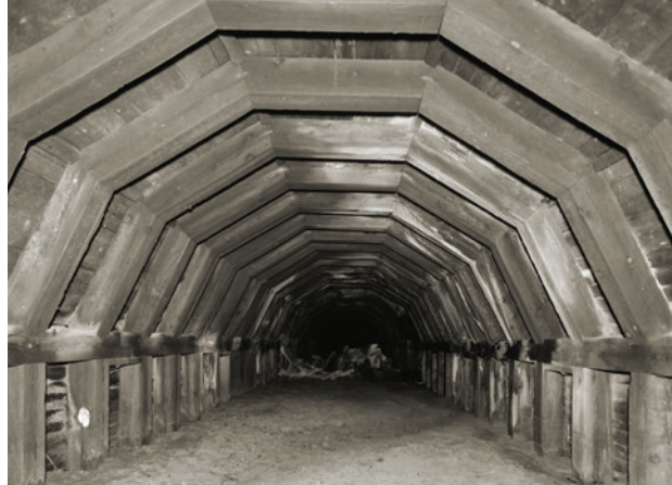
A visit to the nightmarish tunnels beneath Portland, Oregon.
